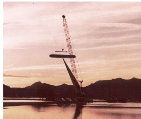
Installation of 40 foot RCS Pole at RATSCAT
