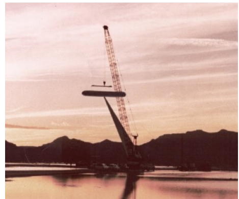
Installation of ogive RCS pylon at RATSCAT
